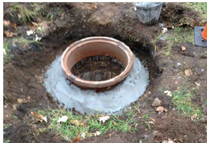
Infiltration & Inflow Repairs
