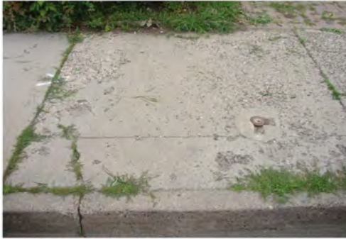
Deteriorated Sidewalk
