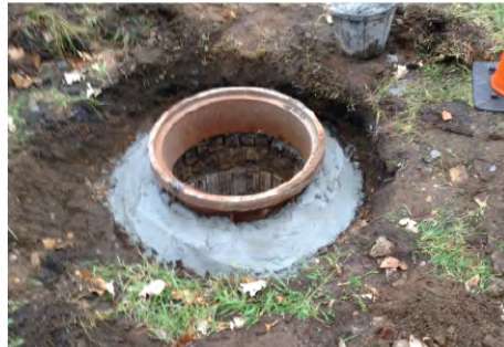
Infiltration & Inflow Repairs
